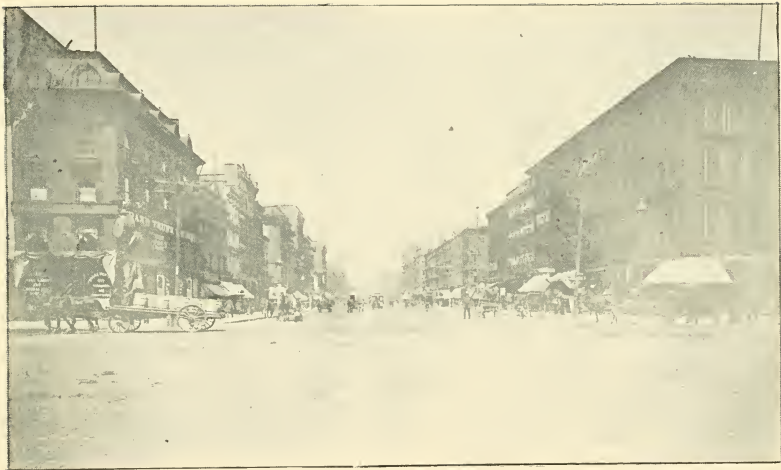
STREET VIEW, LOOKING NORTH ON WOODWARD AVENUE, FROM JEFFERSON AVENUE.
